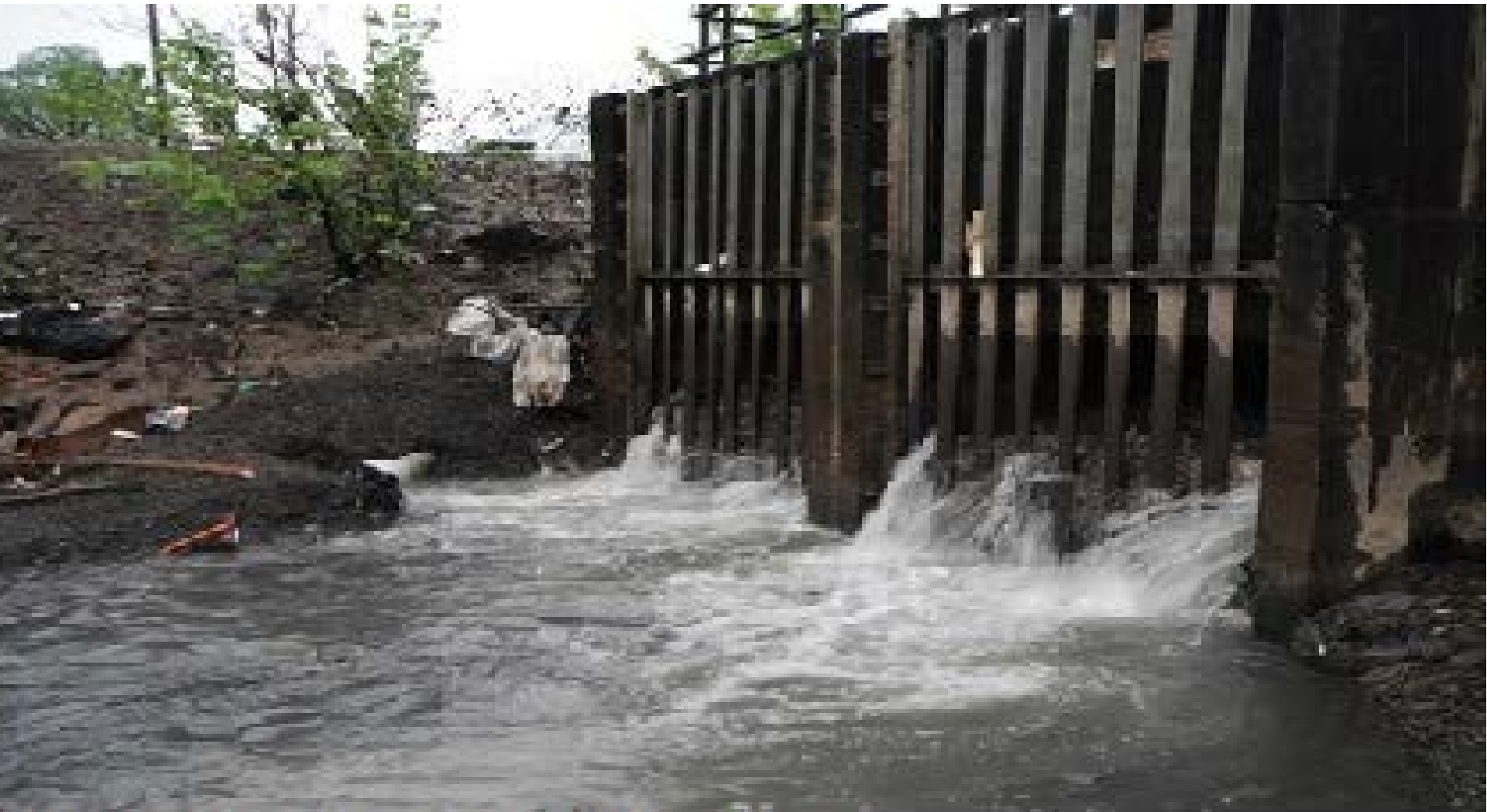
Combined Sewer Overflow, Photo credit: EPA
