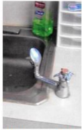
Old Classroom Bubbler
