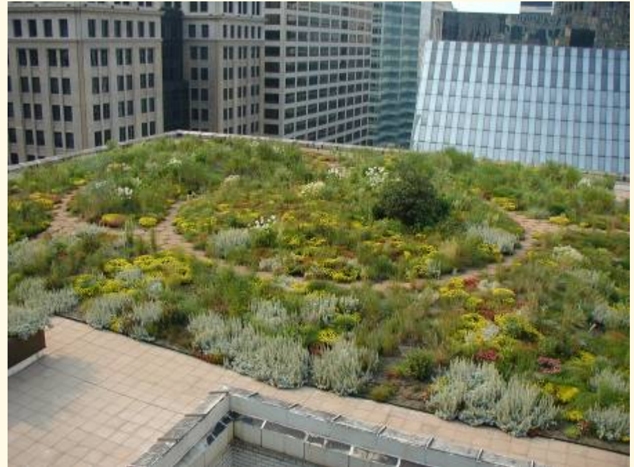
Chicago City Hall Green Roof. Photo courtesy of Roofscapes, Inc.
